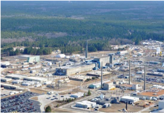
Fig. 1. SRS HB-Line Nuclear Processing Facility
